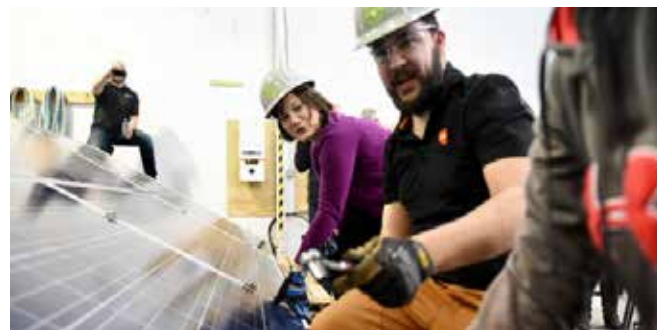
Minister Shannon Phillips helps install solar panels at Gridworks Solar Energy Training Centre
