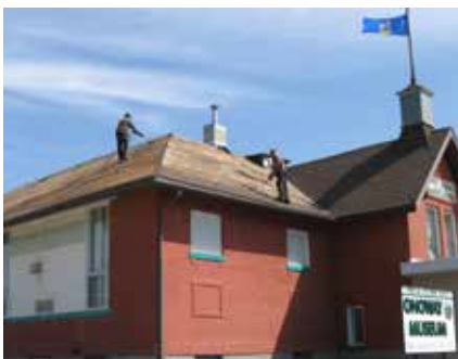
Re-shingling of the roof on the Onoway Museum (originally Beaupré School built in 1921)
