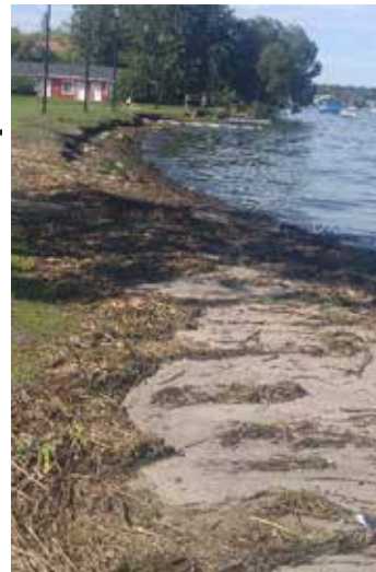
Damage to Public Beach
